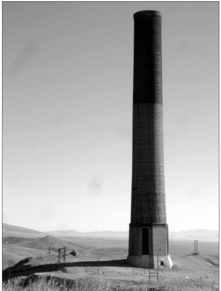
Anaconda's stack stands 585 feet, 1 1/2 inches on Smelter Hill.
